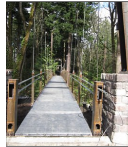
The new Ravine Bridge at BBG
